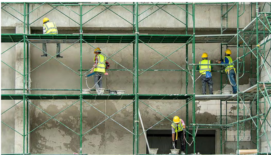
Use of scaffolding for facility maintenance
