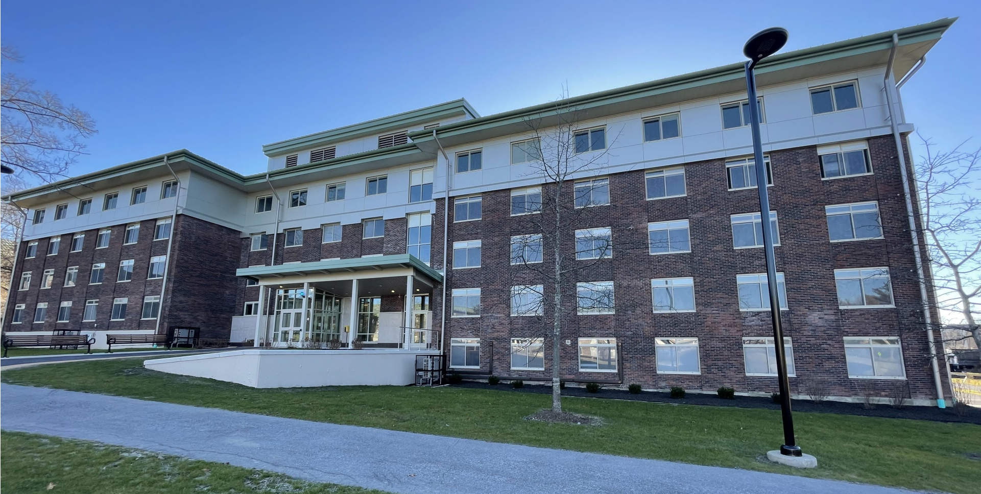
New Paltz : Awosting Hall : Design – Architecture Plus : Construction – Consigli Construction (CMR)
