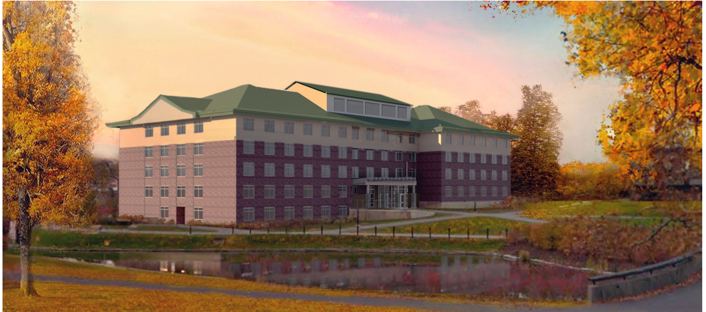
New Paltz : Mohonk Hall : Design – Architecture Plus : Construction – Consigli Construction (CMR)
